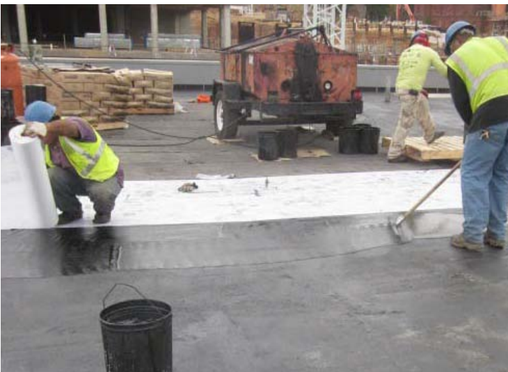
Crews installing hot rubberized asphalt.
