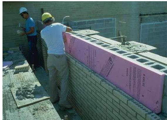
**Figure 6: Mortar Bridging**
