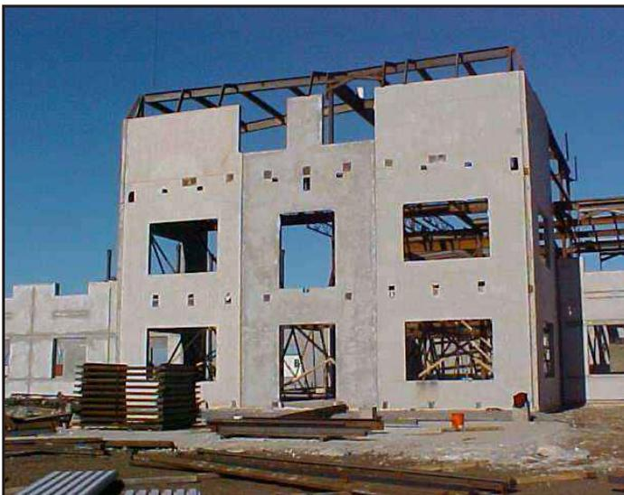
The architectural side is the outside face of the wall. The exterior layer at the Sydney Home for Special Care is three inches thick and include “reveals,” which are decorative indentations molded into the outer surface. At the Sydney home, reveals were two per panel and three-quarters-of-an-inch deep. They will be painted in a different color than the rest of the exterior surface.
