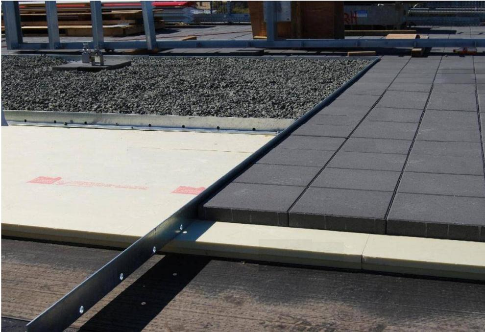
Commonly referred to as “ upside down , *irma* or *prma* roofs ” this method of insulated roofing simply means the insulation is placed above the waterproofing membrane and held in place by a specified ballast , usually river pebbles or concrete pavers.
